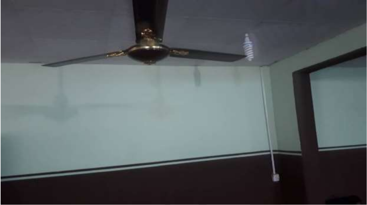
Figure 13: Electrical rewiring in Hall 3 Common Room
