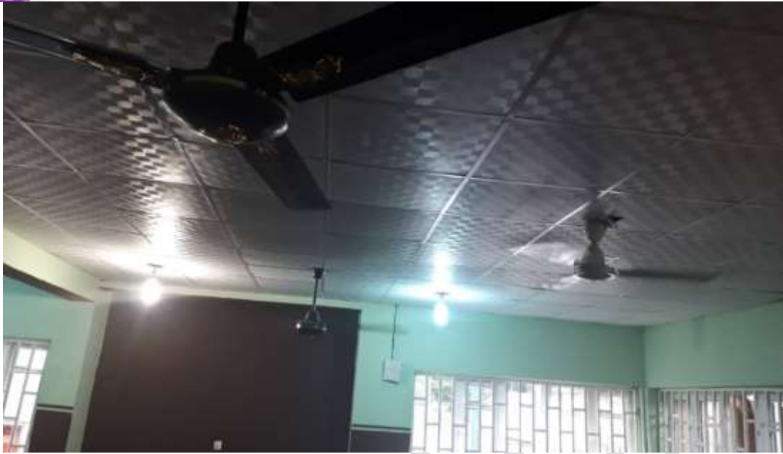
Figure 9: Newly installed ceiling and fans in Hall 3 Common Room
