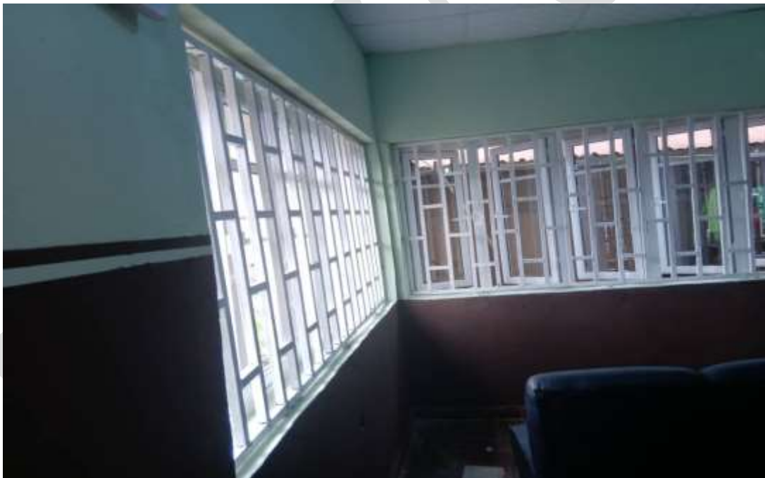
Figure 8: Newly installed window protector at Hall 3 Common Room
