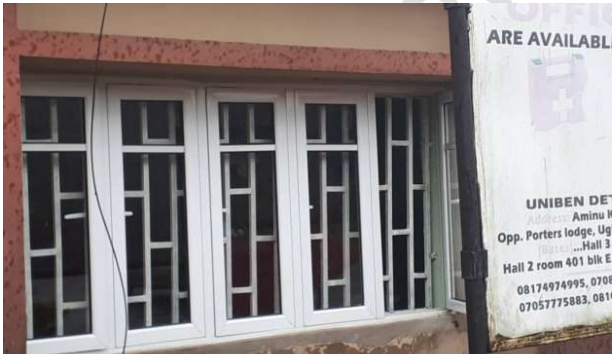
Figure 6: Newly installed window frames at Hall 3 Common Room (1)
