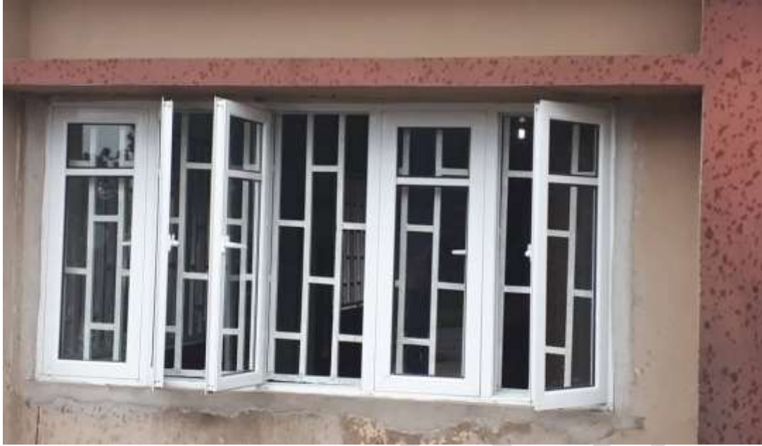
Figure 7: Newly installed window frames at Hall 3 Common Room (2)
