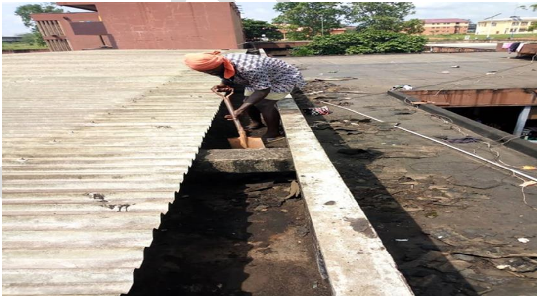
Attachment 8: Clearing of failed bituminous surface of roof
