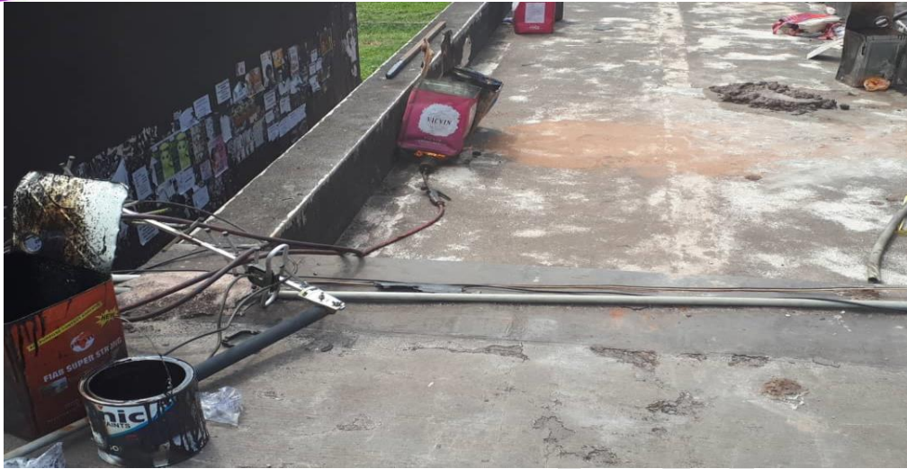
Attachment 9: Heating of bitumen for roof repair
