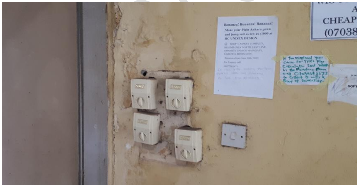
Plate 6: Hall 1 Small Reading Room before Repair (2) – Notice dampness as a result of leaking roof
