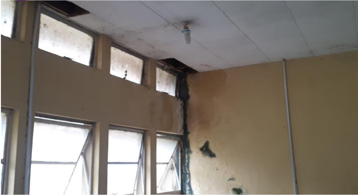
Plate 5: Hall 1 Small Reading Room before Repair (1) - Notice dampness as a result of leaking roof
