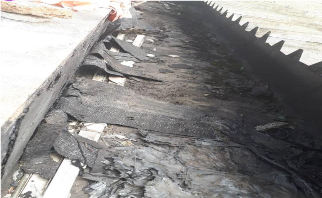
Plate 8: Roof of Hall 1 Reading Room (Failed Bituminous felt) – this makes the roof to leak
