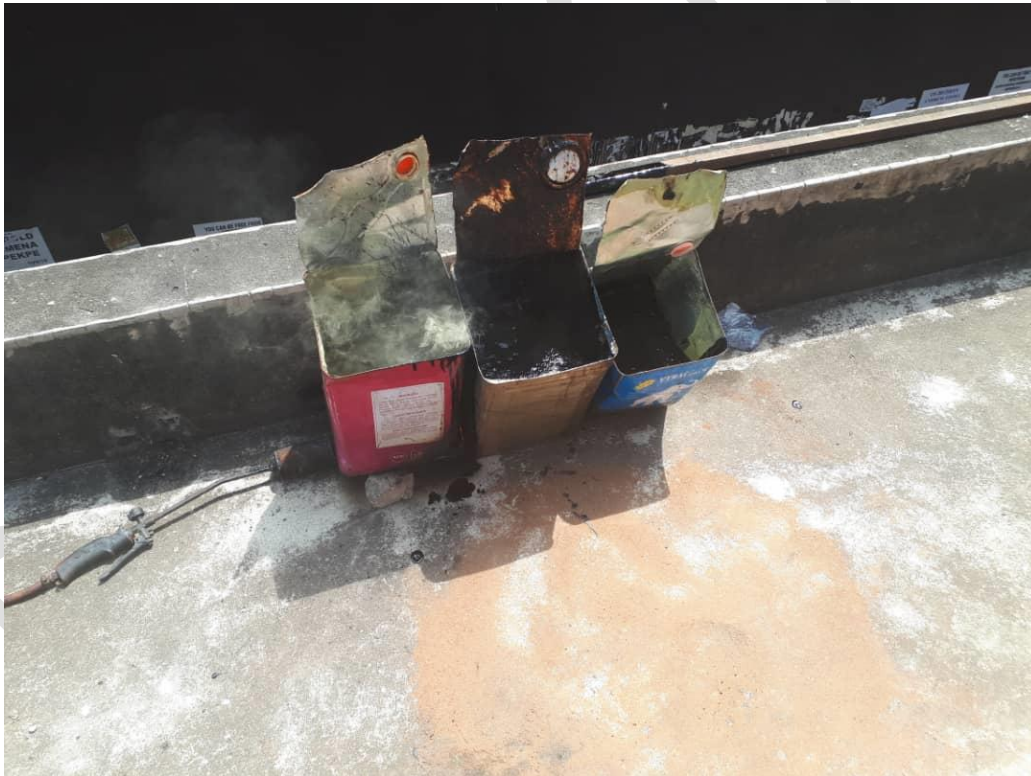
Attachment 10: Heating of bitumen for roof repair (2)
